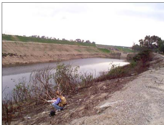
EXISTING DOMINGUEZ GAP
